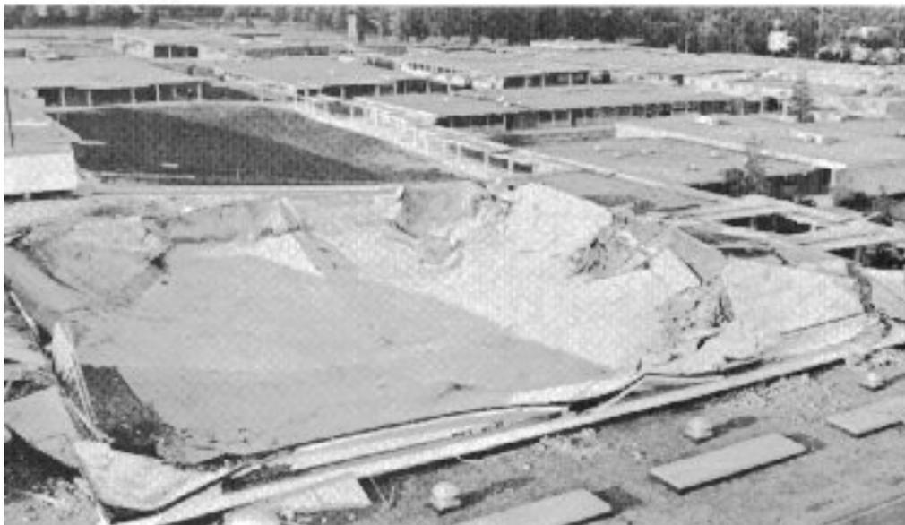
Figure 1. Newspaper photograph of the collapsed hyperboloid shell [1]
