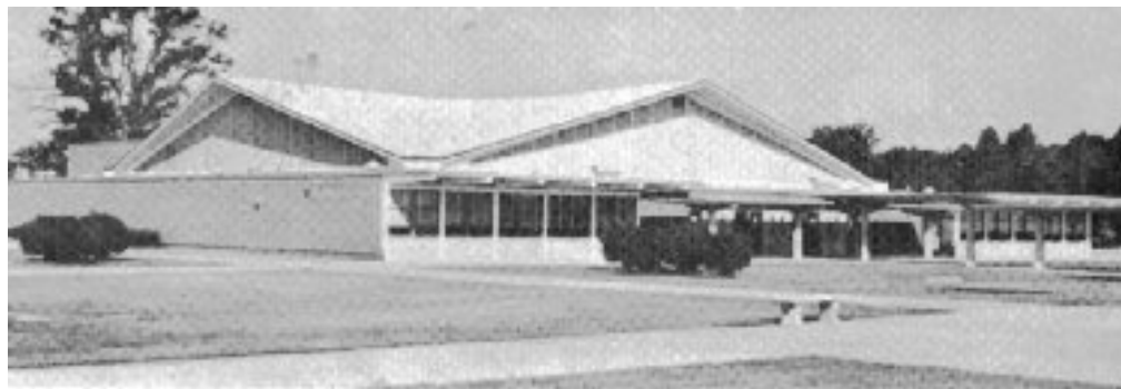
ipped roof gymnasium was one of four identical structures designed by same firm.
